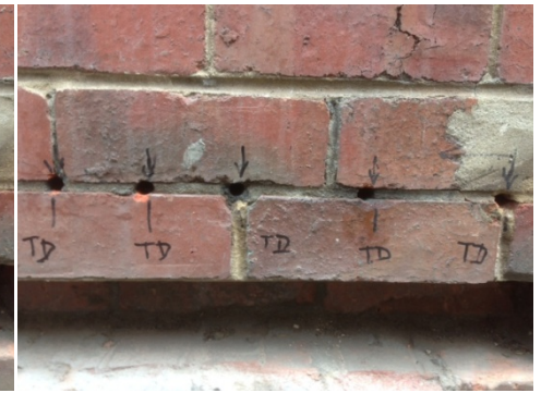
After 48hrs: curing
